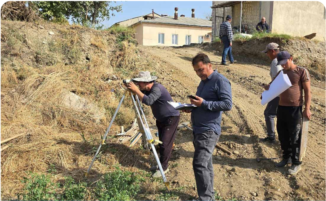
Construction site for biological treatment infrastructure at Dehmoy Hospital, Tajikistan
